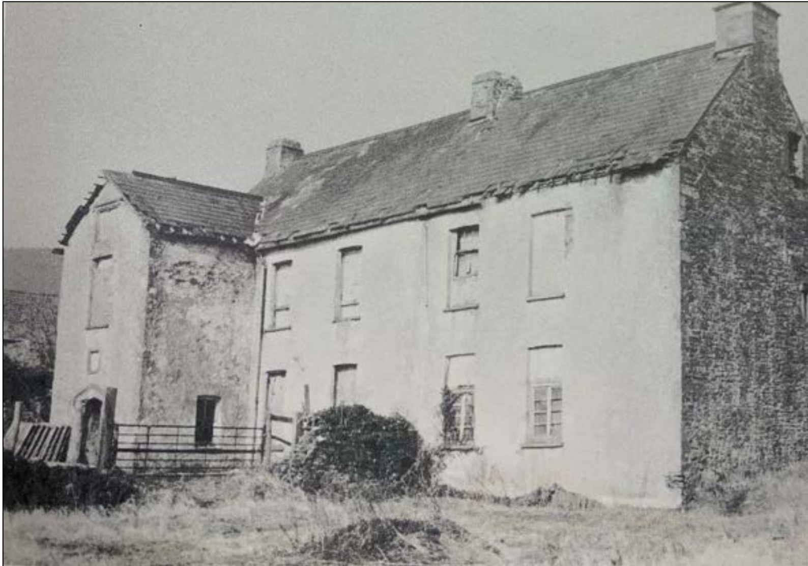
Plate 38. Blaen Baglan House, from E. Jones' Baglan Then and Now A Pictorial Record
